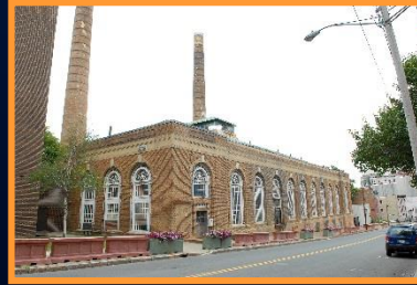
Sheridan Power Plant, Albany 77,350 sq. ft. 104 years
