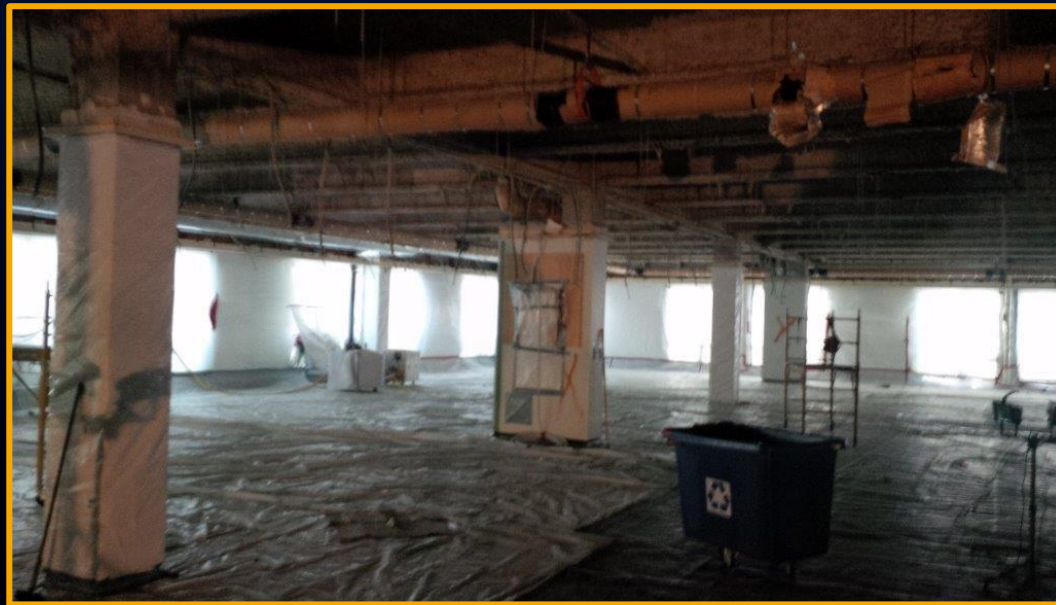
Example: Asbestos Abatement Project on P1 Level of Empire State Plaza
